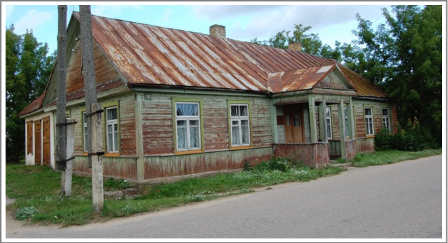
Little green house once owned by a Dumesh.
